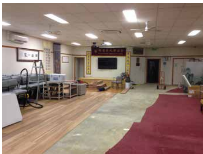
New floor coverings, part of the renovation work, 2017.
