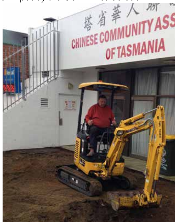
Front entry renovation, 2017.
